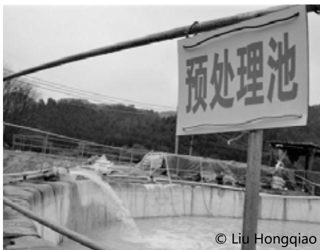
A pre-treatment pool at a mine site. These pools are a requirement of China's new environment standards
