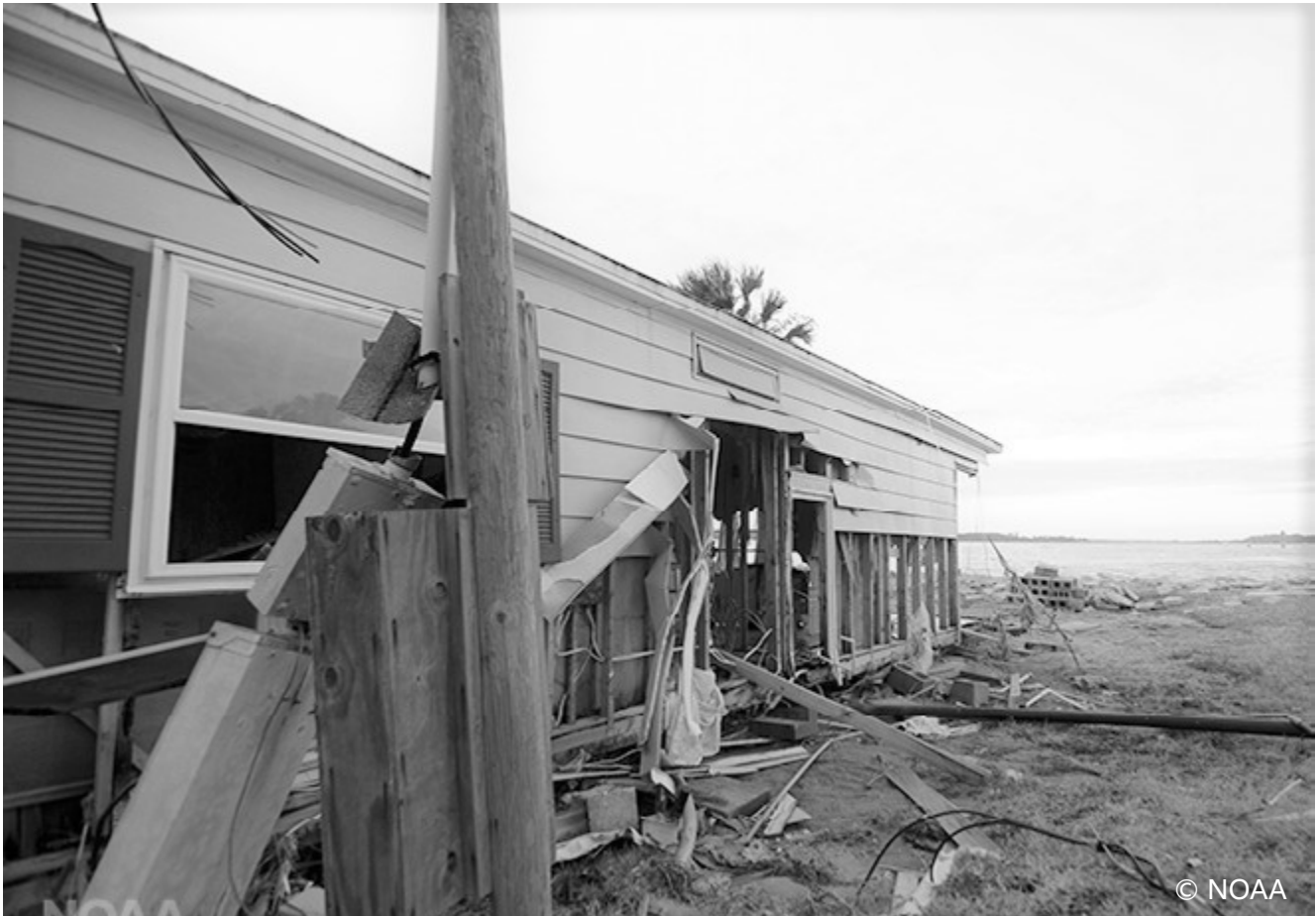
Damage from Hurricane Matthew last year. Cutting help for people and communities struggling with climate change impacts is just one area where the budget is looking to save money
