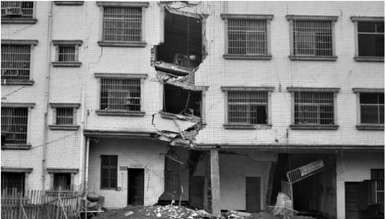
Large numbers of building in Lengshui, Hunan, are dangerous due to subsidence caused by mining. In 2015, a building in the township of Duoshan split down the middle
