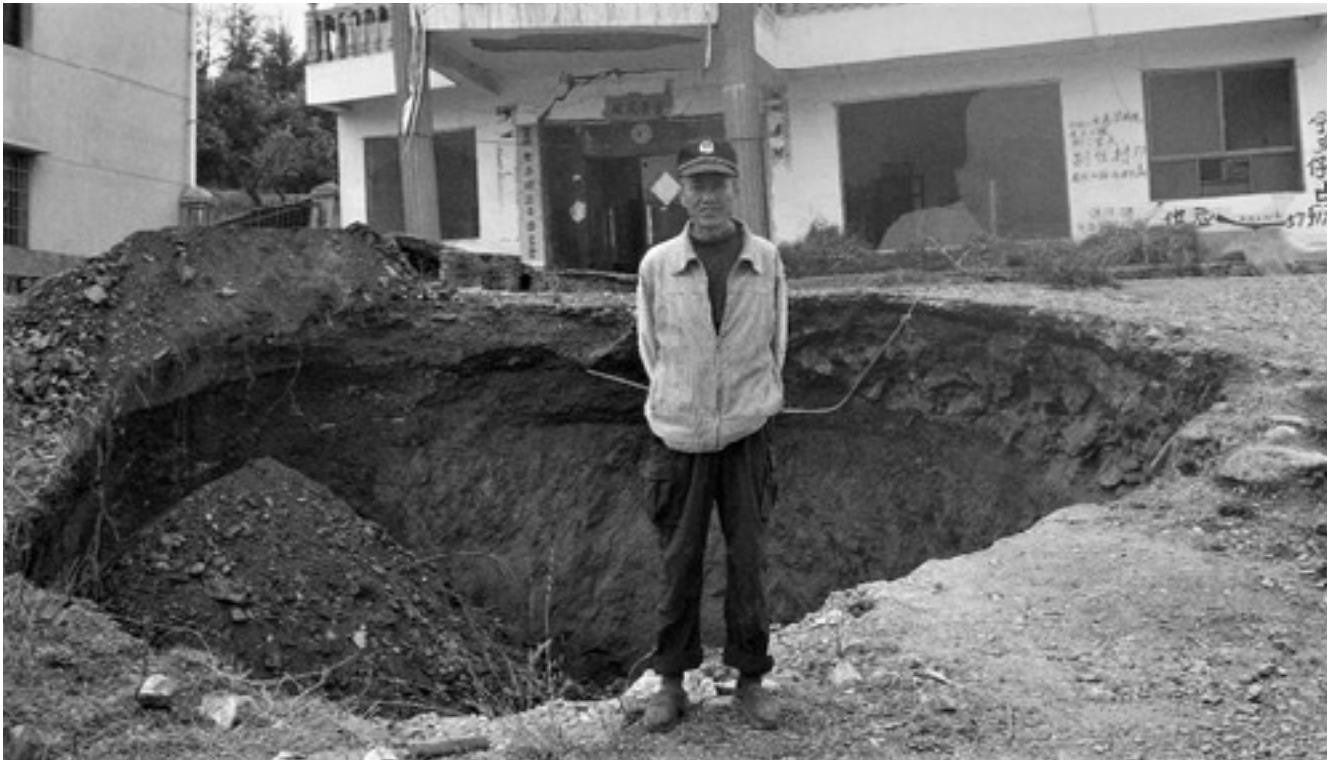
In 2007, Ouyang Shican used his life saving to build a modern home of several hundred square meters for his family. Soon after they moved in the foundations started to subside and walls cracked, a deep hole appeared
