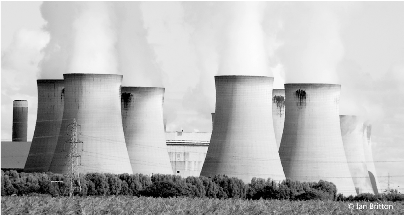
The Drax coal-fired power station in northern England where the owners have withdrawn from a planned CCS project
